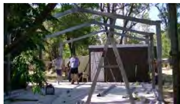
Above: The frame is being sorted, bolted together and then erected.
